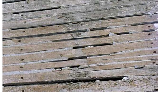
Split lathe wall with plaster removed. Individual boards are nailed to the stud then plaster is applied over. Usually studs and lathe were not level and the professional plaster ensured level walls.
