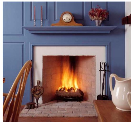
A Rumford fireplace in a colonial home. They are marked by a shallow firebox, which increases heating efficiency.
