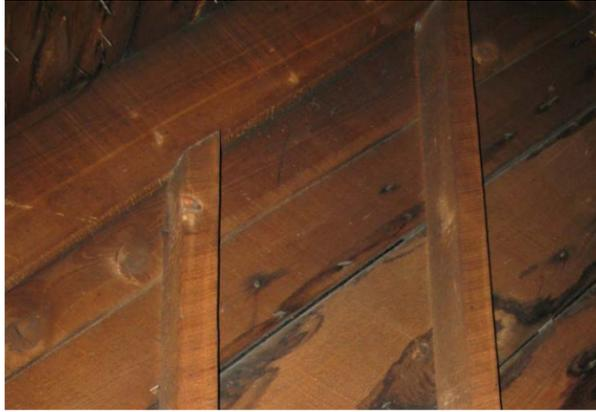
Circular saw marks found on a balloon frame house and visible in the attic. Look for framing in your basement and attic when not easily accessible on main living levels.
