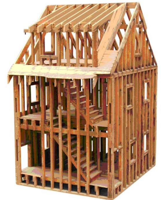
*Balloon framing construction detail. This method of building made construction quicker – using prefabricated elements (such as studs and joists). It is easily identifiable by two story studs and was common through the nineteenth century.*
